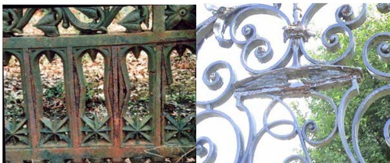
Fig. 1 – Ornamental parts damage exposed to atmospheric corrosion.
